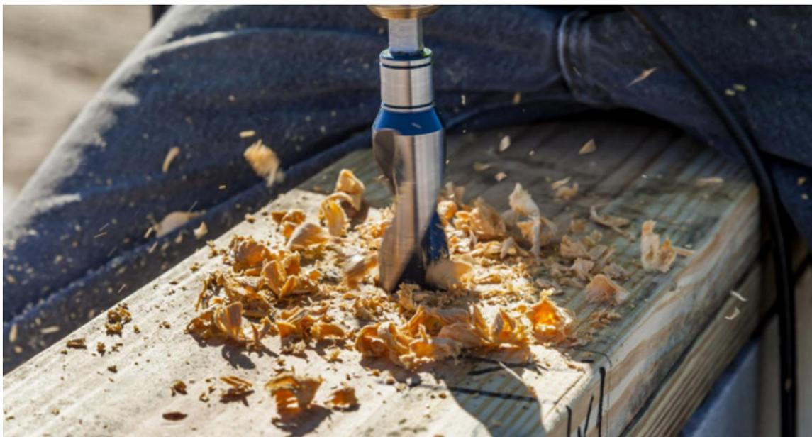
**Figure 28.** Drill a Hole above each Anchor Bolt
