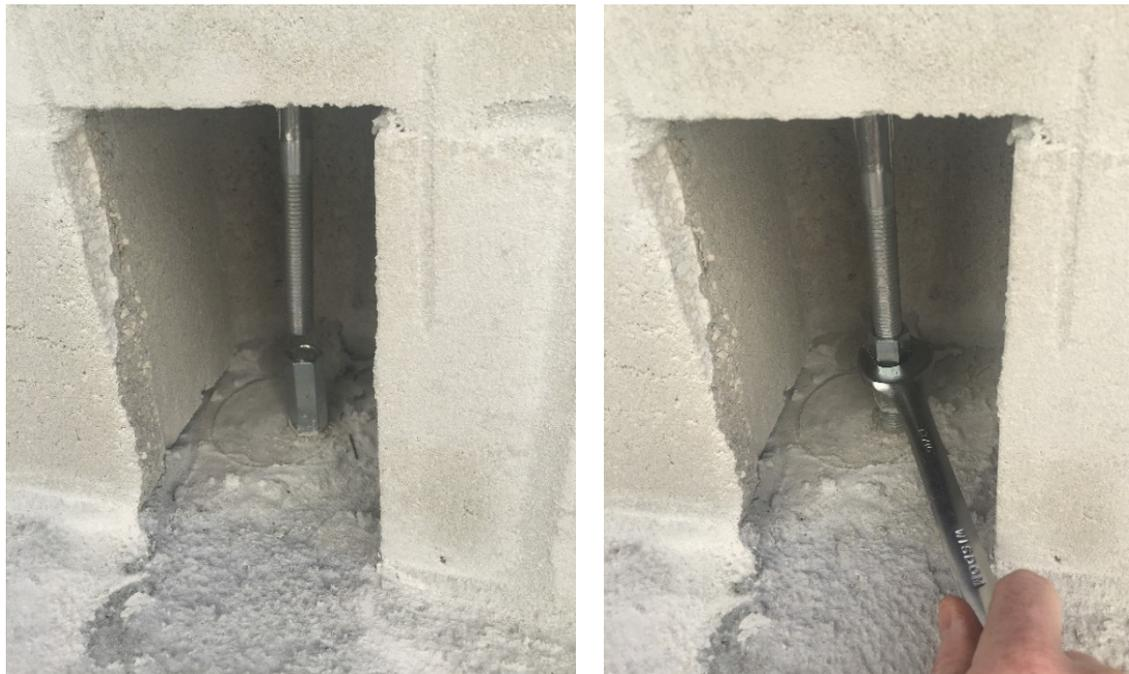
**Figure 20.** Connecting the Cable to the Anchor Bolt
