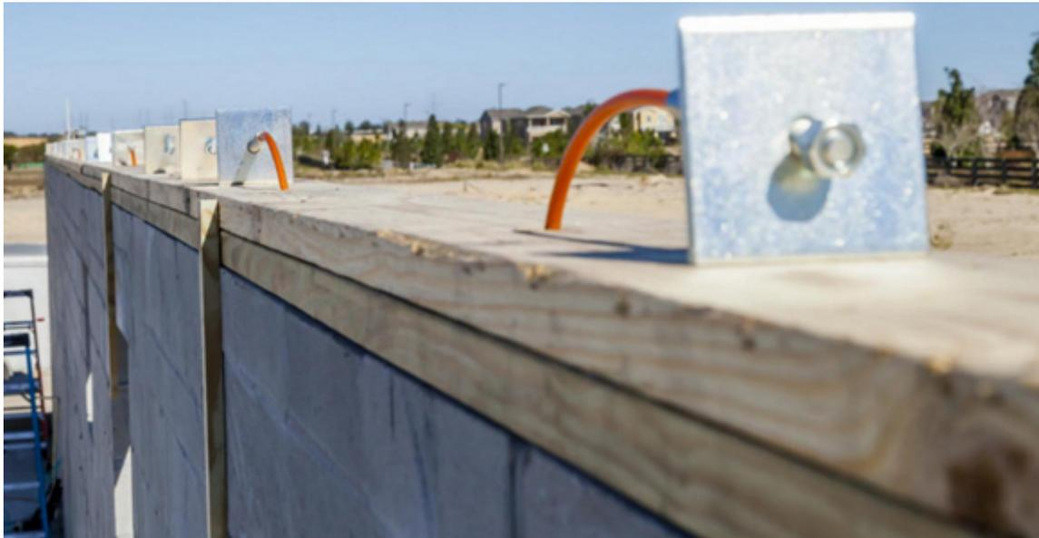
**Figure 29.** Feed each Cable through the Holes
