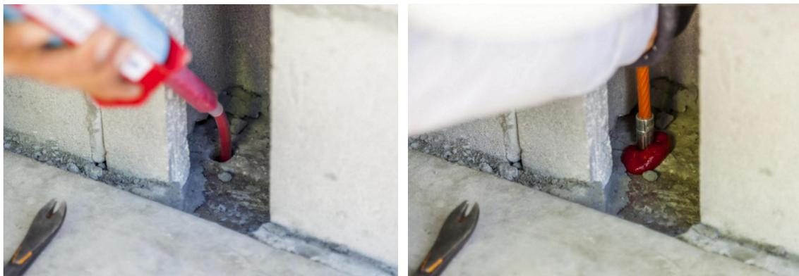
**Figure 30.** Fill the Anchor Hole with Epoxy
