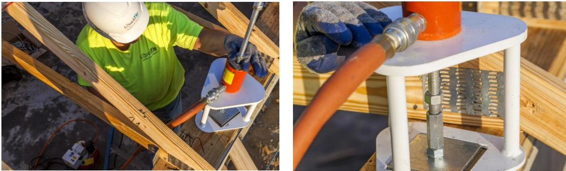
**Figure 22.** Tension the Cables to the Specified Load
