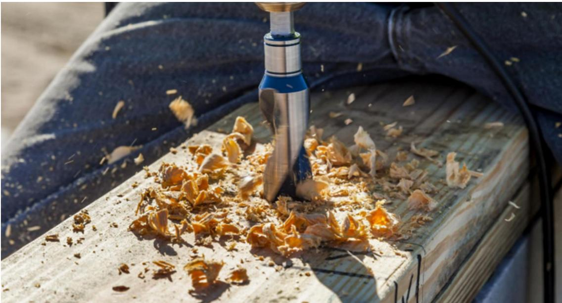
**Figure 18.** Drill a Hole Above Each Anchor Bolt
