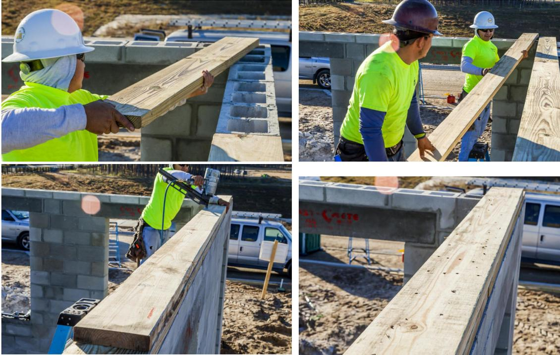
**Figure 27.** Install Double Top Plate
