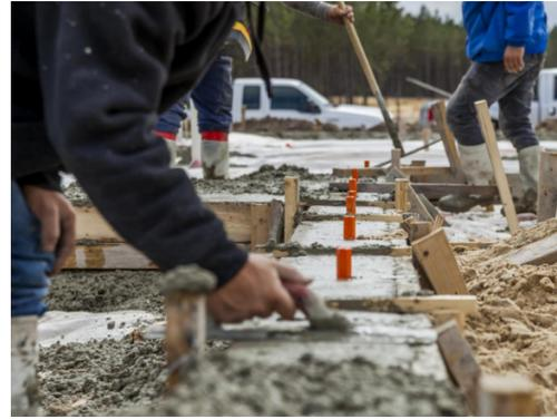
**Figure 24.** Fill Foundation Forms with Concrete
