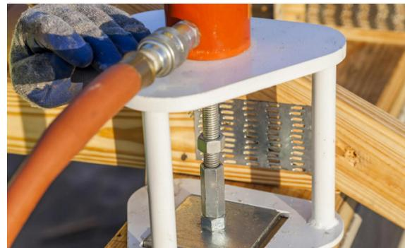
**Figure 32.** Tension the Cables to the Specified Load
