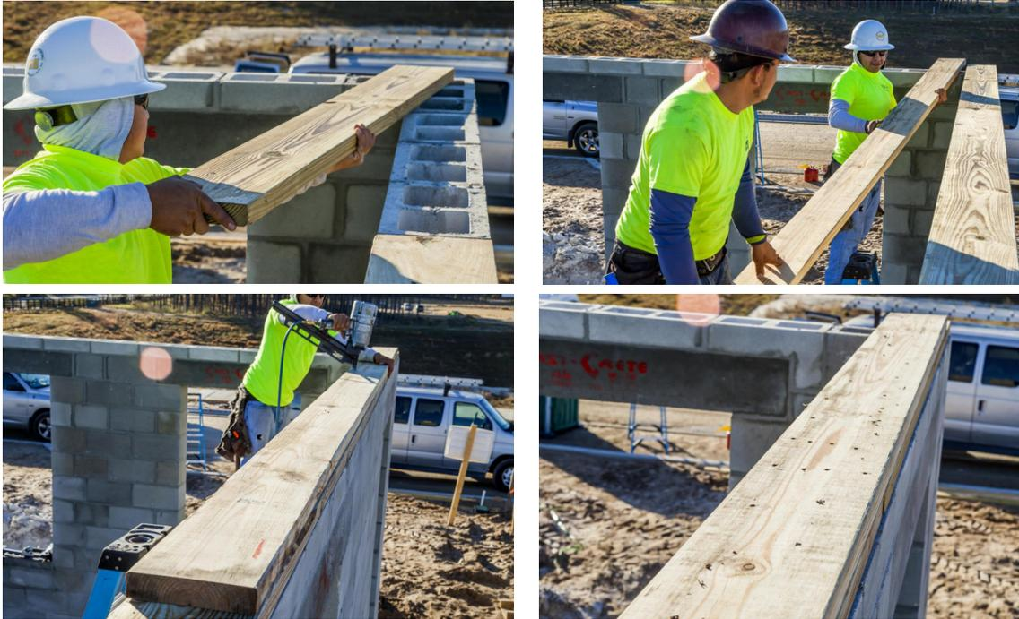
**Figure 17.** Installation of the Double Top Plate
