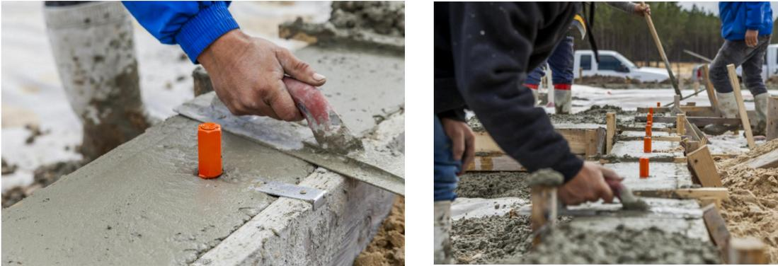
**Figure 15.** Fill Foundation Forms Around the Anchor Bolts
