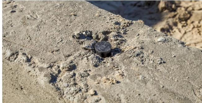
**Figure 25.** Backing out the Anchor Bolt and Capping the Hole
